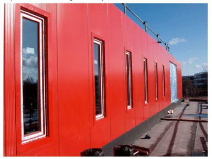
Load-bearing behaviour of Openings with windows acting as a frame?
